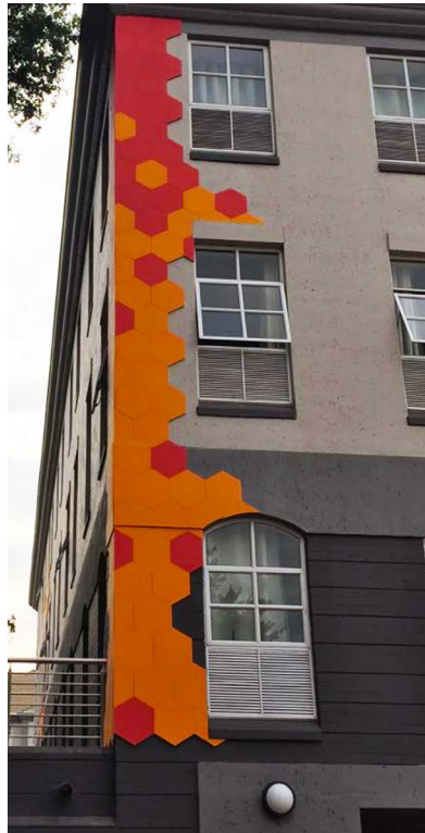
Special tile shapes waterjet cut from 10 mm Nutec Flat Sheet.
