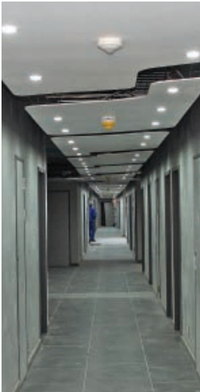
Student Residence Accommodation Waterjet cut 9 mm Nutec Ceiling Board.
