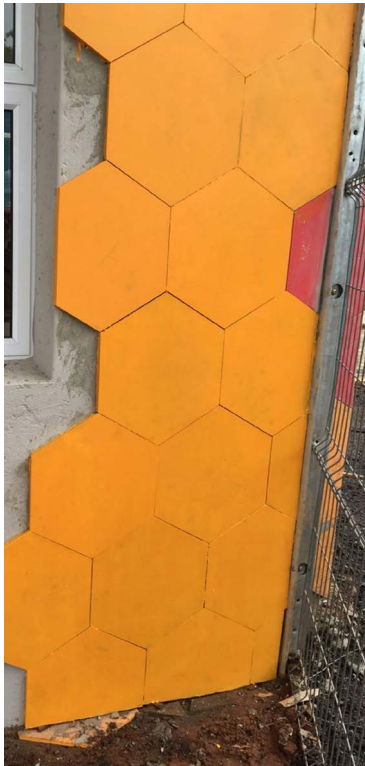
Special tile shapes waterjet cut from 10 mm Nutec Flat Sheet.
