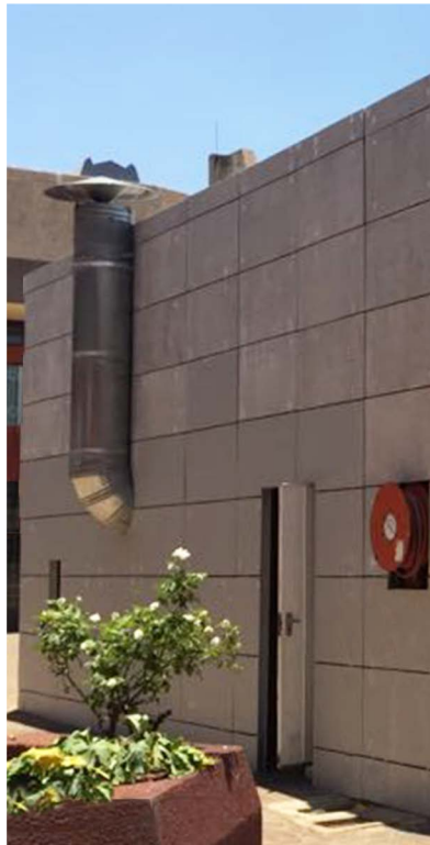
10 mm thick Nutec Flat Sheet Waterjet cut to fit exact apertures and staggered curves to facade.
