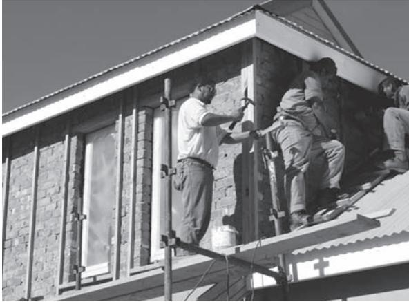
Supporting timber structure used on masonry walls should not be less than 38 mm x 38 mm.
